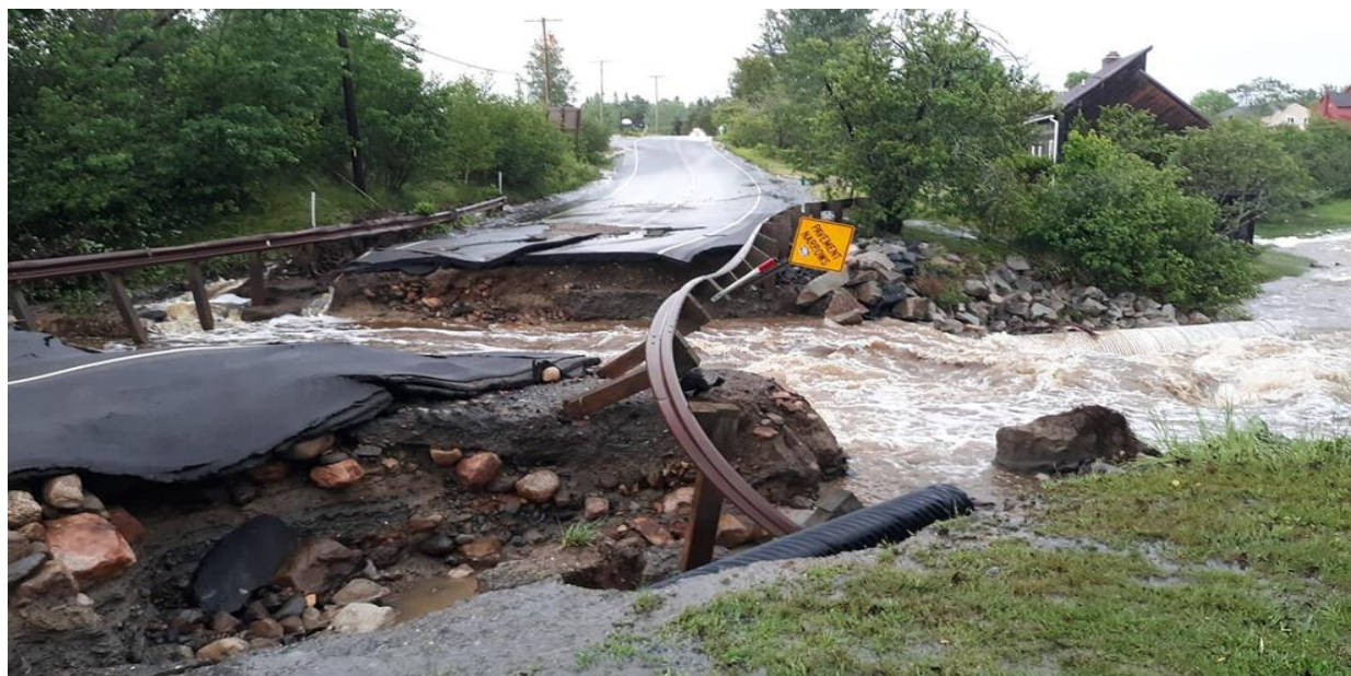
Figure M-1. Birch Harbor Bridge, June 2021
