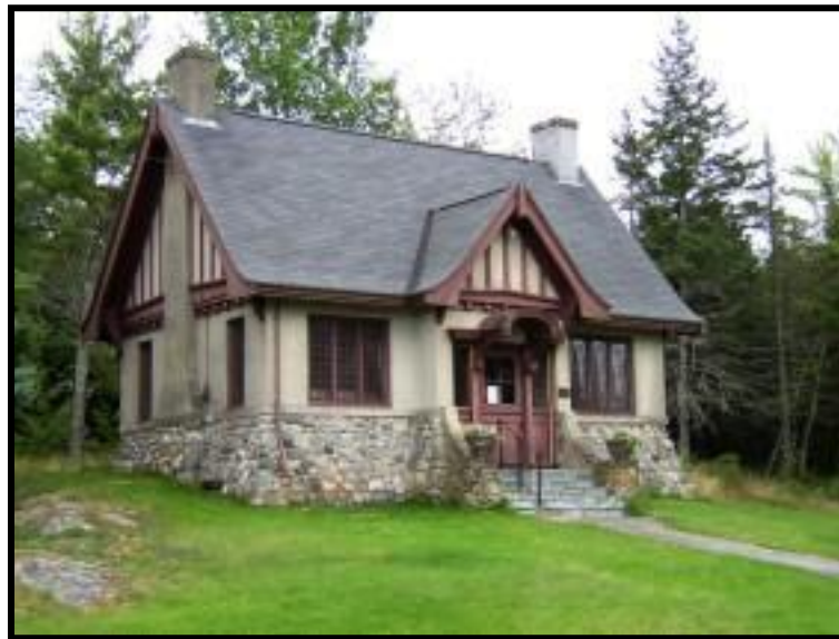
West Gouldsboro Village Library, Route 186
