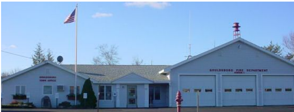
Figure-XX; Gouldsboro Town Office, Fire Station #1
