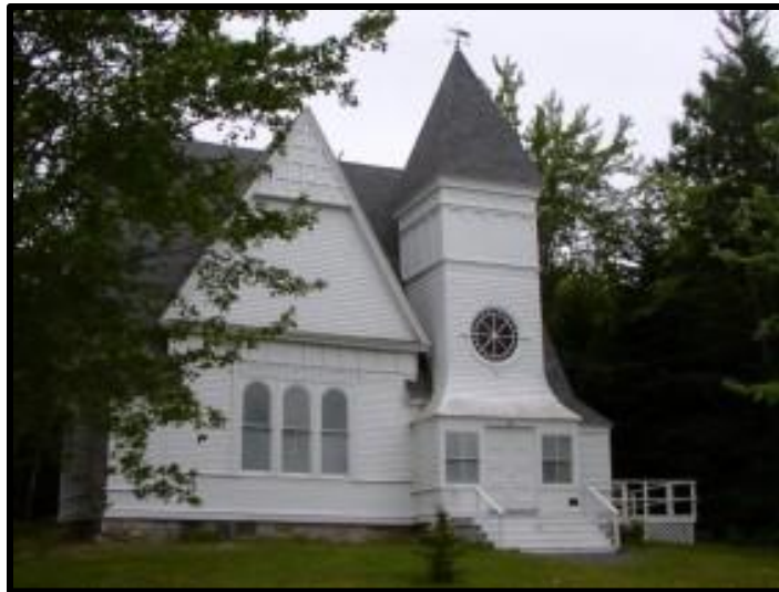
Figure A-4: West Gouldsboro Union Church, Route 186
